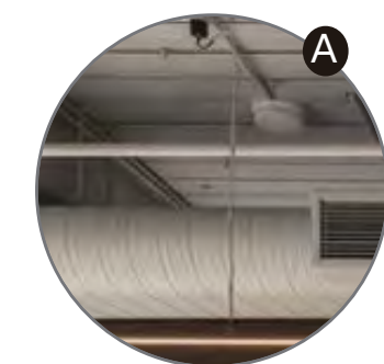
Open Ceiling Sprayed Ceiling
